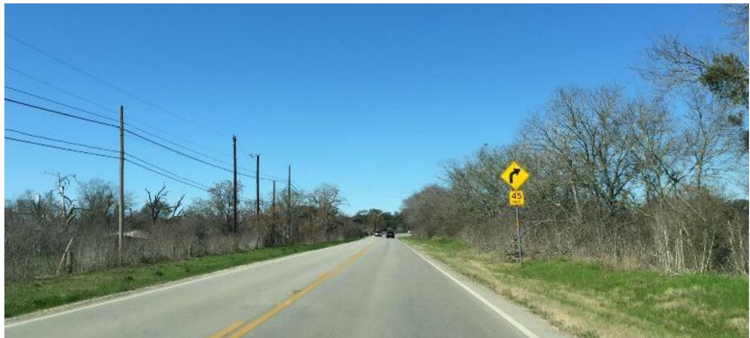
Exhibit 33. Horizontal curve with a posted (advisory) speed of 45 miles per hour and inferred speed 52 miles per hour
